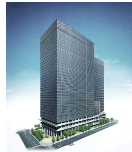
Otemachi 2-chome Area 1st Class Urban Redevelopment Project (Tokyo)
